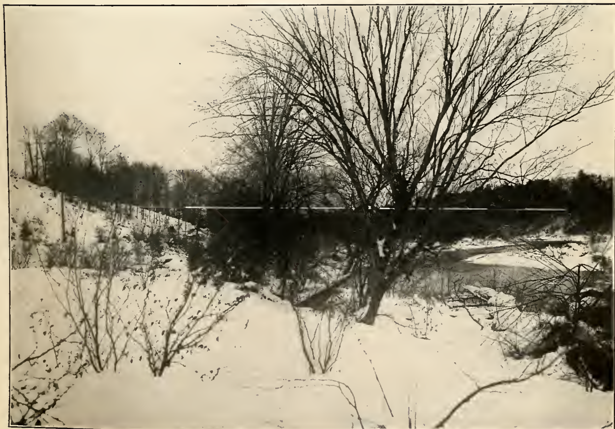
NORTH BRANCH FRENCH CREEK, PA., DECEMBER, 1910. View down stream, showing crest of proposed dam.
